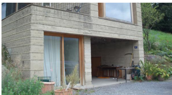
5 Clay House, entrance ground floor through the garage
